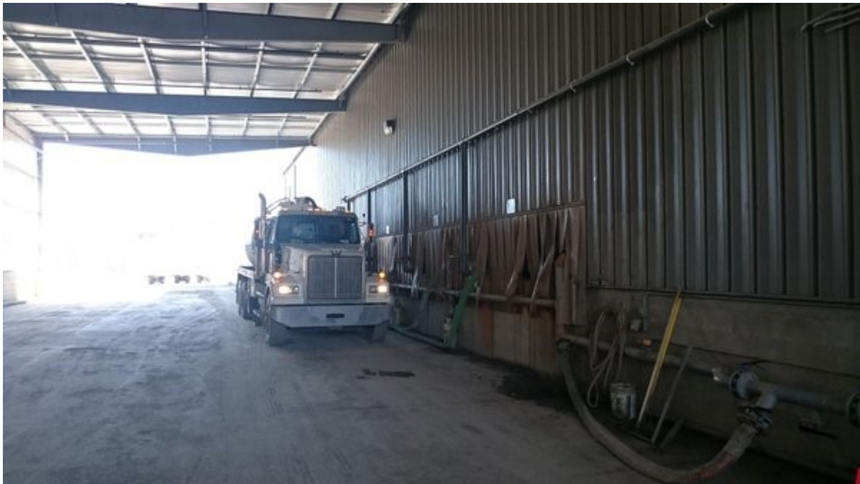
Fig. 1 - Truck offloading waste water in the administration bay of the Eureka Resources Standing Stone Gas Well facility
